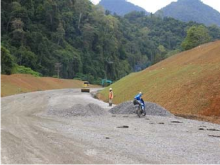
Slope Erosion Protection Lhoong
